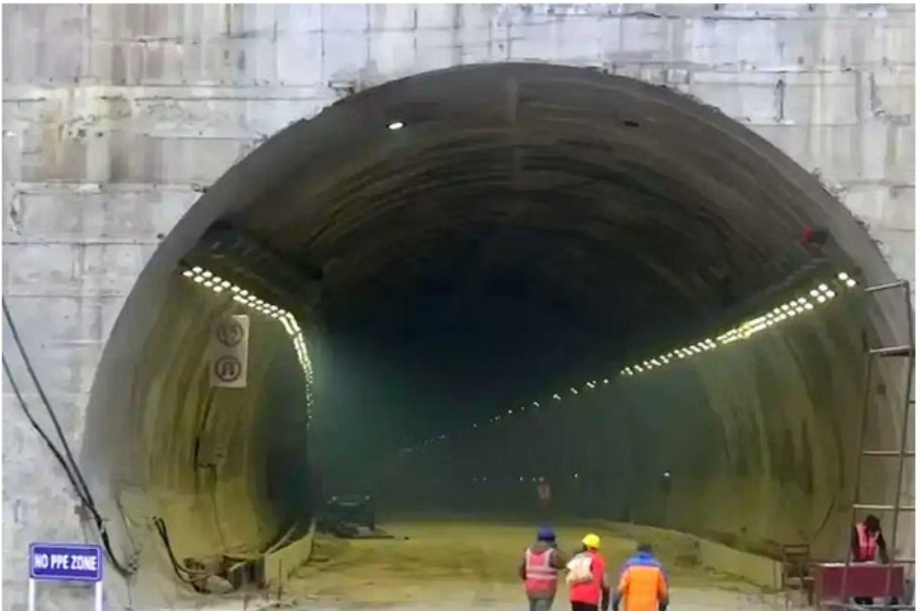
A representative image of a tunnel.
