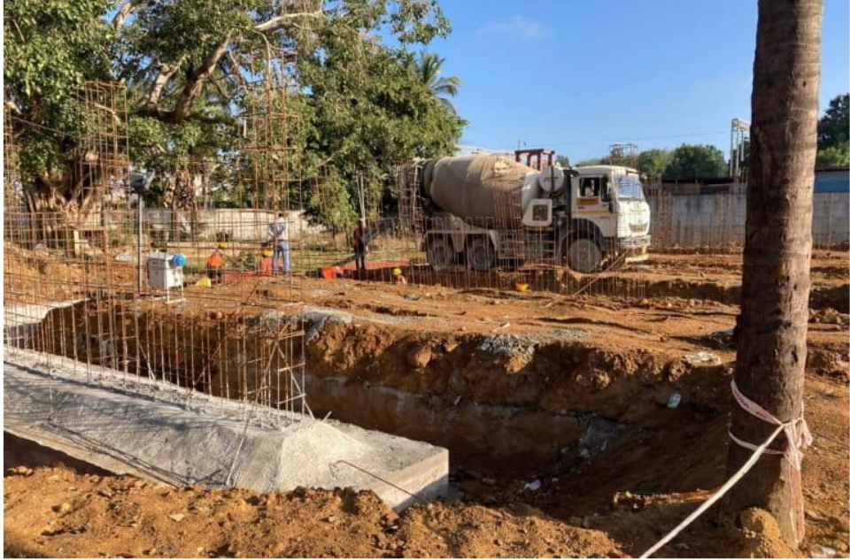
The tunnel also faces a specific vulnerability: its entrance sits in a flood-prone location. Image by Soheli Sarkar.
