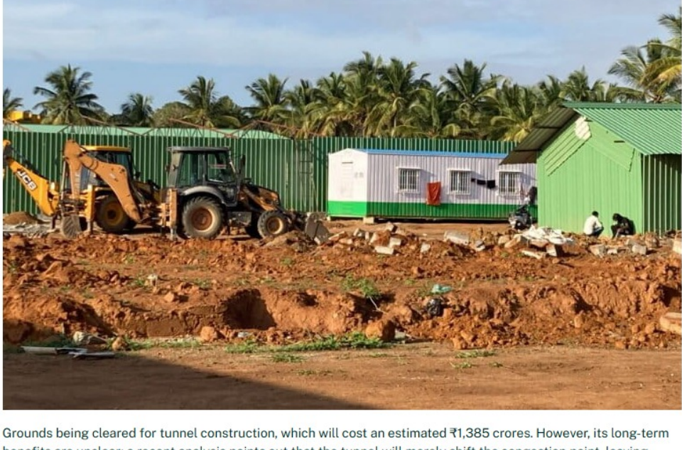
Grounds being cleared for tunnel construction, which will cost an estimated ₹1,385 crores. However, its long-term benefits are unclear; a recent analysis points out that the tunnel will merely shift the congestion point, leaving bottlenecks at its entry and exit. Image by Soheli Sarkar.
