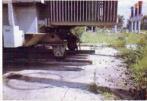
Figure 21. MSEB substation at Umerga.
