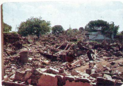
Figure 4. Khilari; Type A structures, grade 5 damage.
