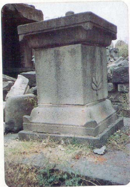
Figure 24. Clockwise rotation of stone block in Kavatha temple.
