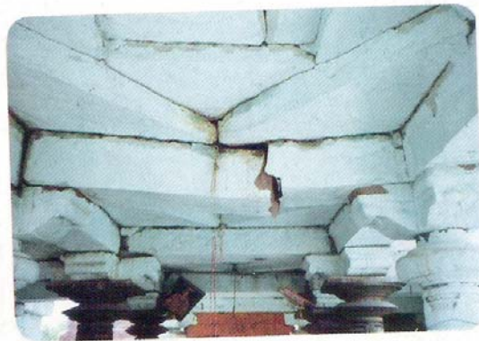
Figure 26. Broken stone beam, Ambabhavani temple, Khilari.
