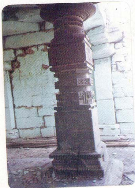
Figure 27. Fractured column, Ambabhavani temple, Khilari.
