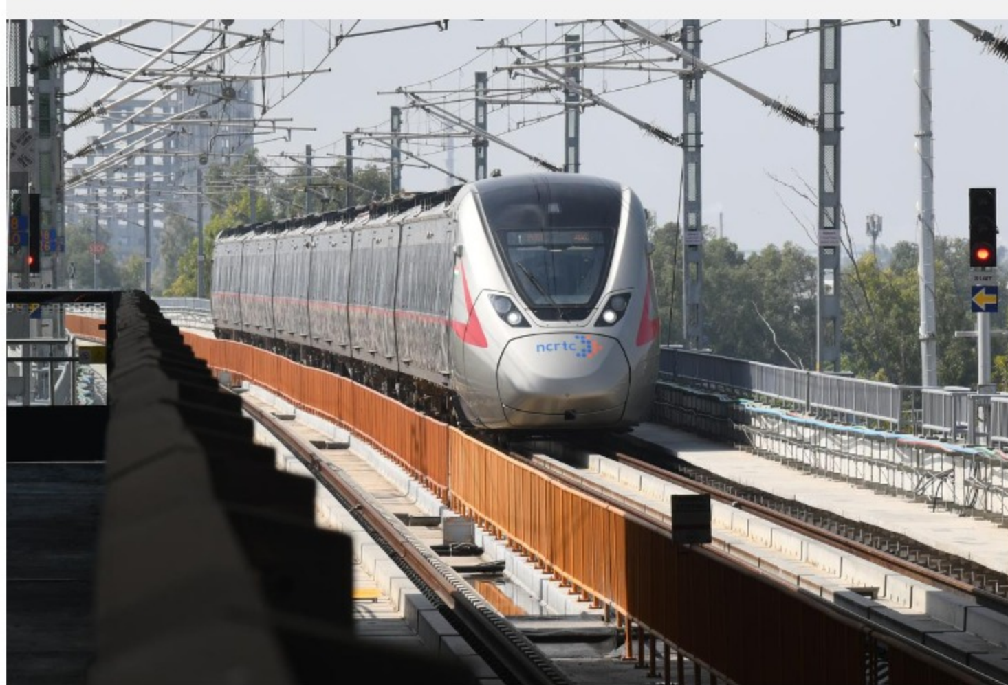
Delhi-Meerut Regional Rapid Transit System (RRTS), in Ghaziabad. | Photo Credit: SHASHI SHEKHAR KASHYAP
