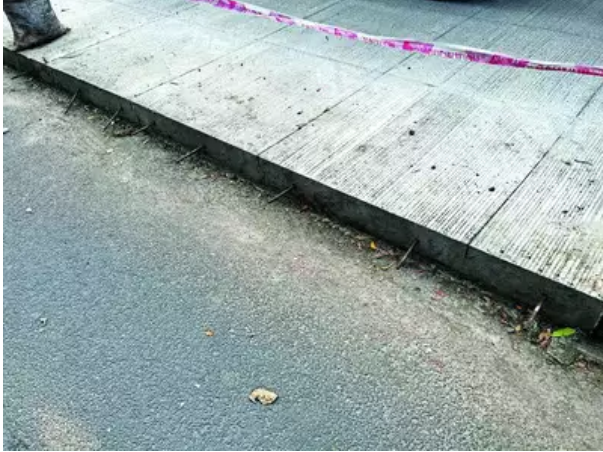
Close up of a whitetopped section in Koramangala.
