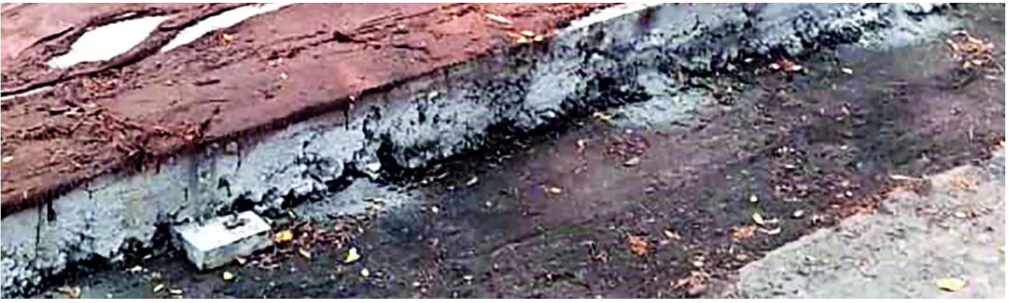
White-topping underway in Malleswaram
