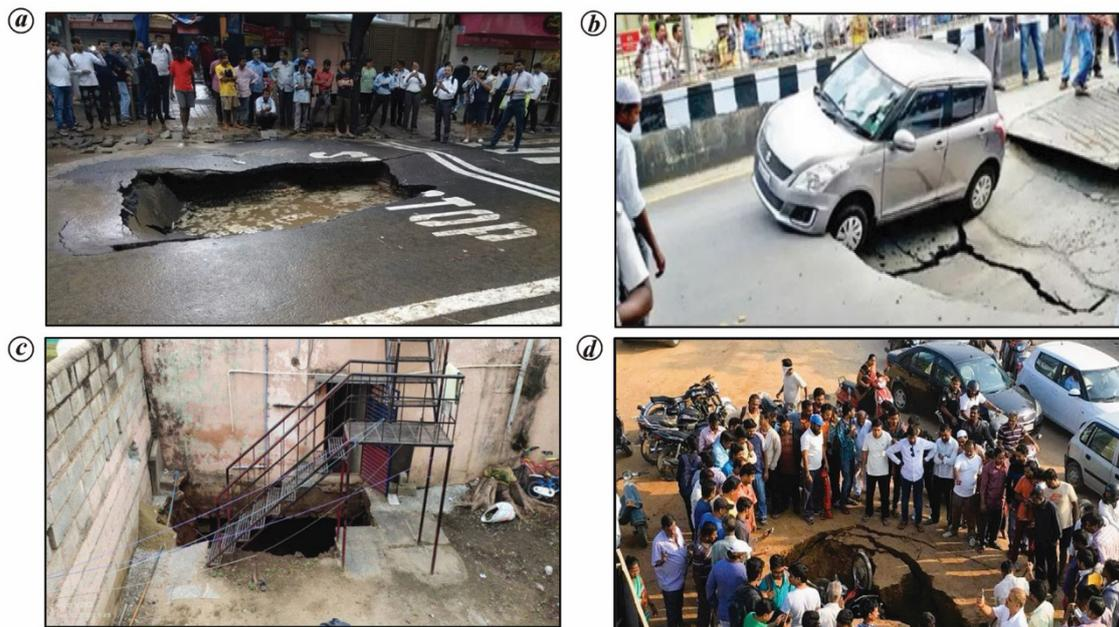
**Figure 1.** Cavity formation incidents due to (a) water pipe burst (26 June 2018, Mumbai); (b) metro tunnelling (2 August 2016, Bengaluru); (c) metro tunnelling (1 October 2021, Bengaluru), (d) improper compaction of subgrade (5 November 2016, Hyderabad).
