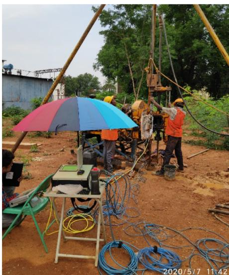
**Fig. 6** Typical photo from the site showing SPT tests and energy measurement
