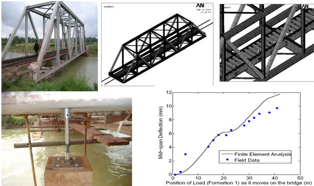
**Figure 40: Details of the truss bridge and finite element model of the bridge with longitudinal and close-up Views, and comparison of measured and simulated quasi-static moving load test**
