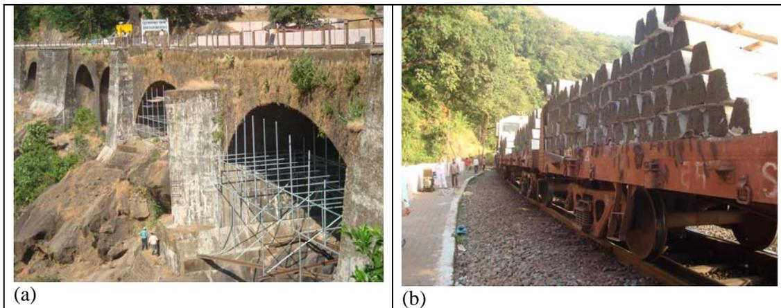
**Figure 41: Condition assessment of a multi-span railway bridge; (a) 5-span masonry arch bridge; (b) sleeper loaded BFR wagons used in static and dynamic load tests**
